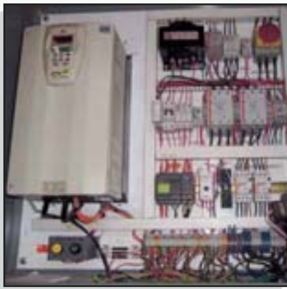
Variable Frequency Drive for smooth operation & drive comfort. Self-troubleshooting PLC control. Relay logic and software redundancy.
